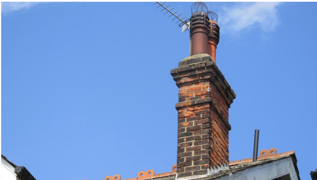
Right Chimney Stack from the front
