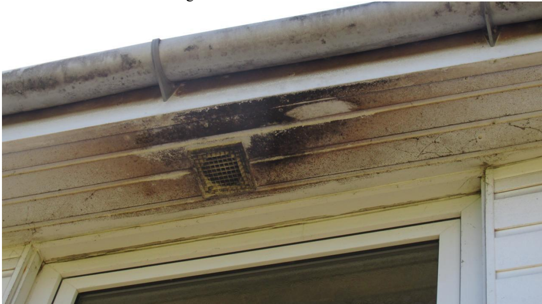
Soffits and barge boards at the front
