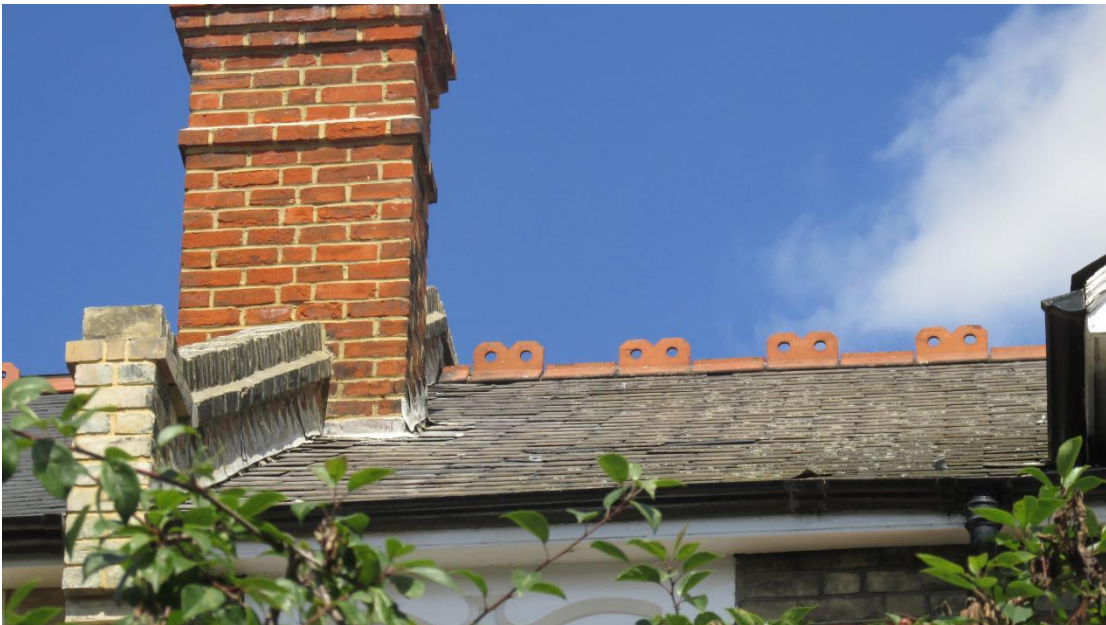
Left chimney stack flashing
