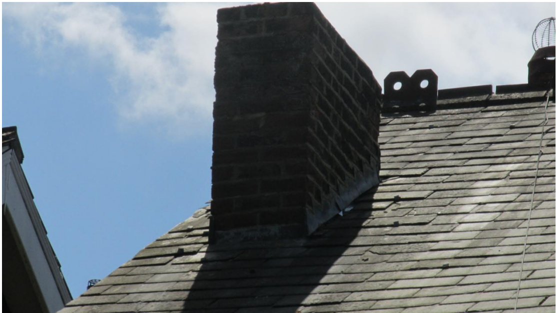
Roof from the rear
