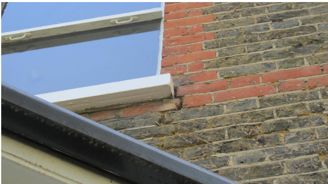
Rear wall above the bay window
