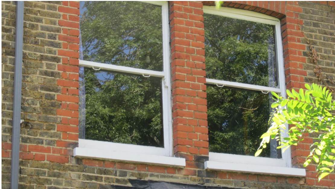
Rear sash timber window
