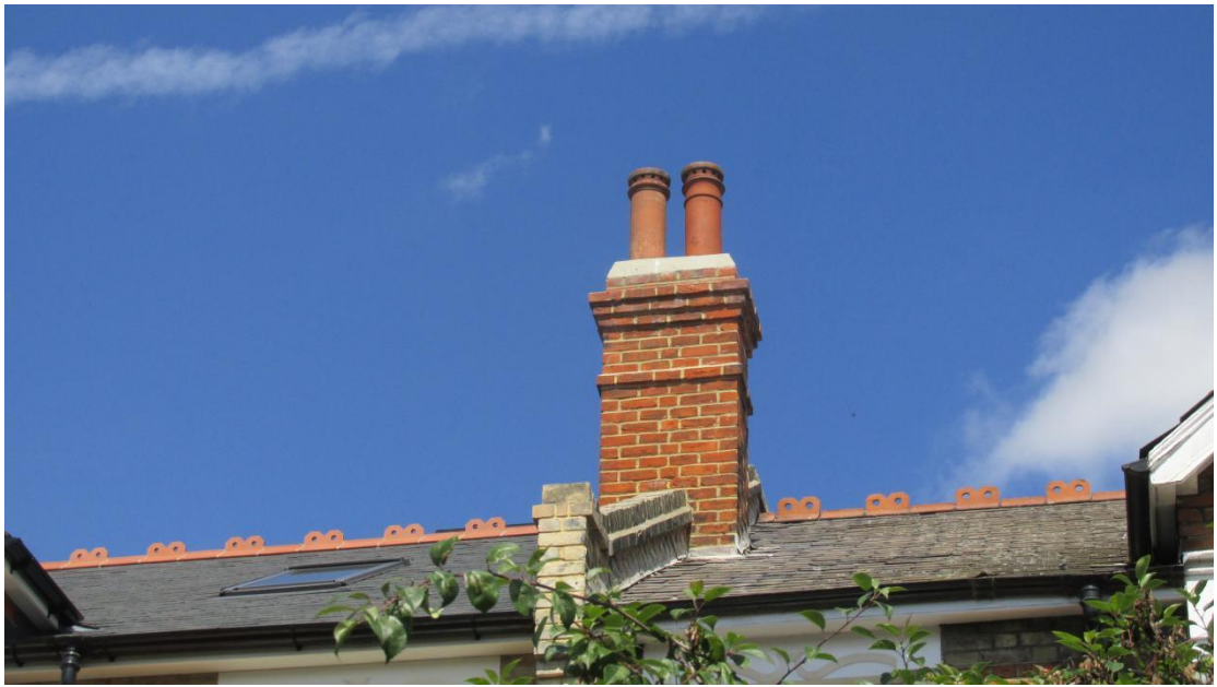
Left chimney stack from the front
