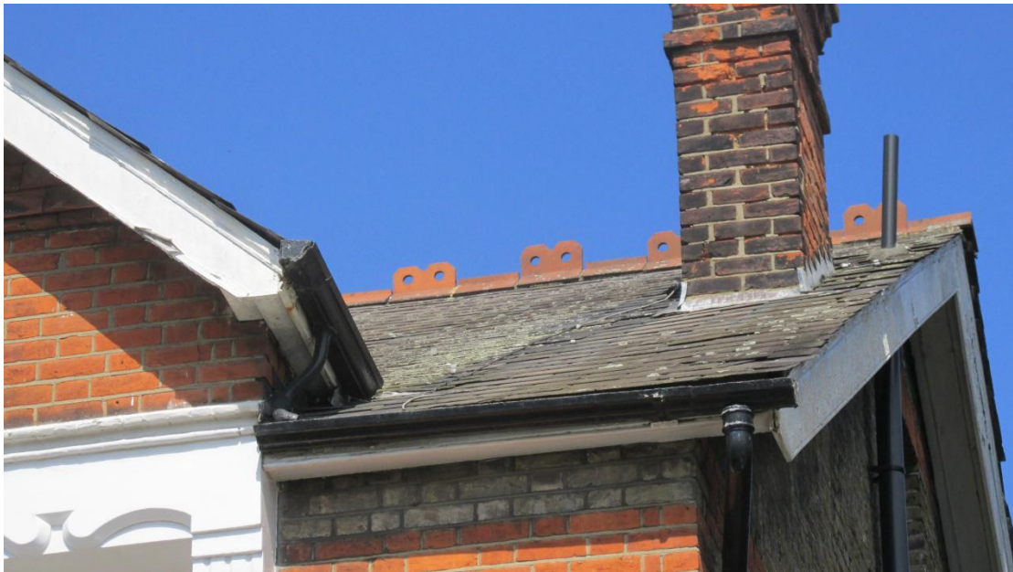
Roof covering from the front right
