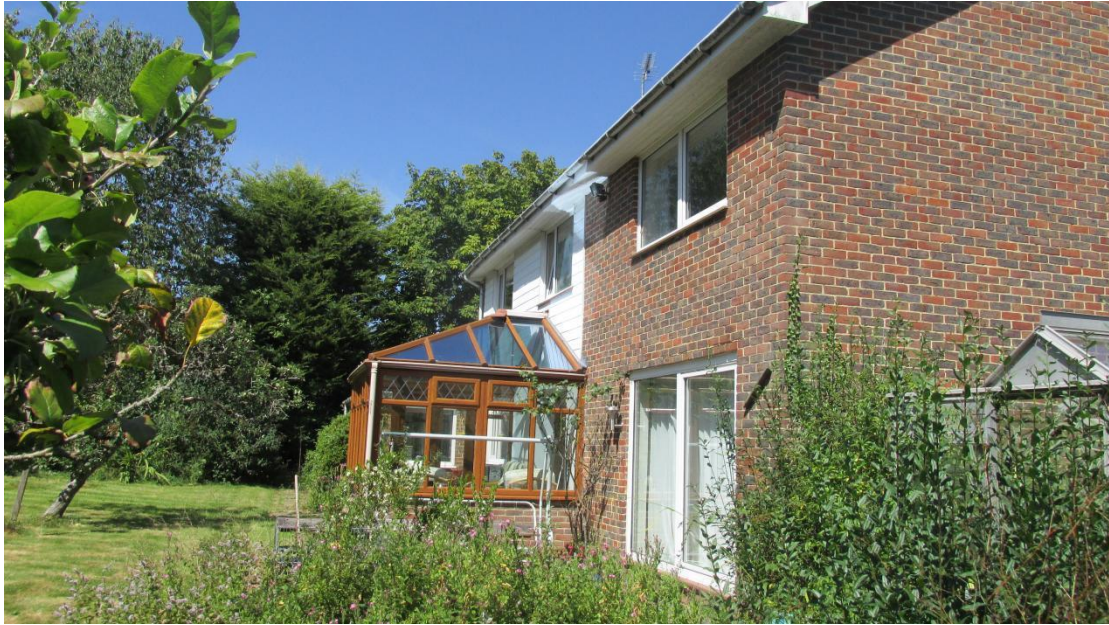
Barge boards and soffits at the rear
