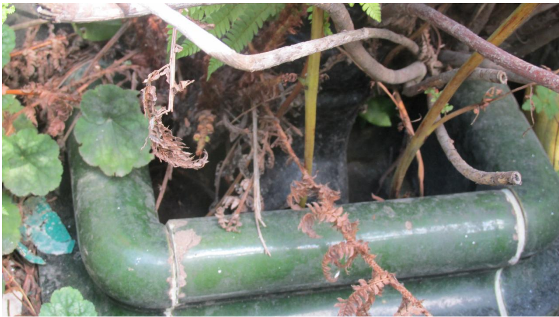
Downpipe gully at the front full of vegetation
