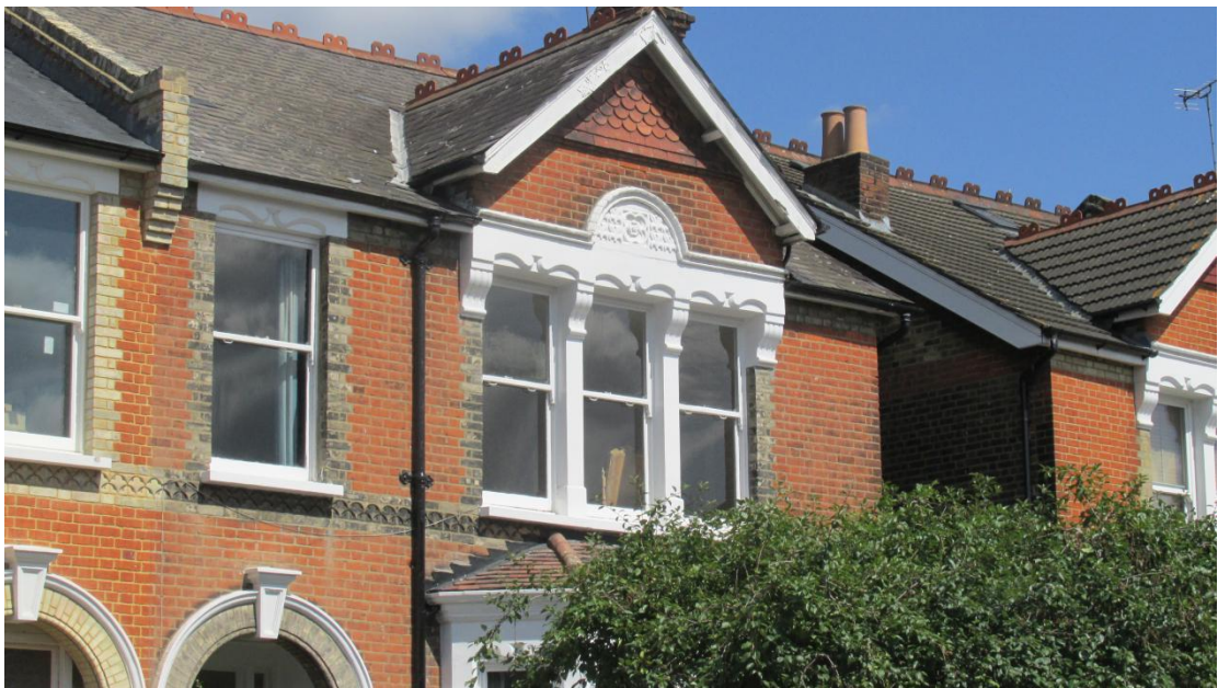
Roof on the front bay window
