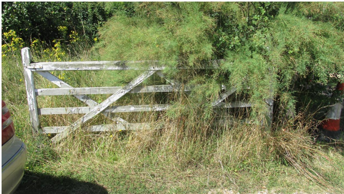
Outside entrance timber gate
