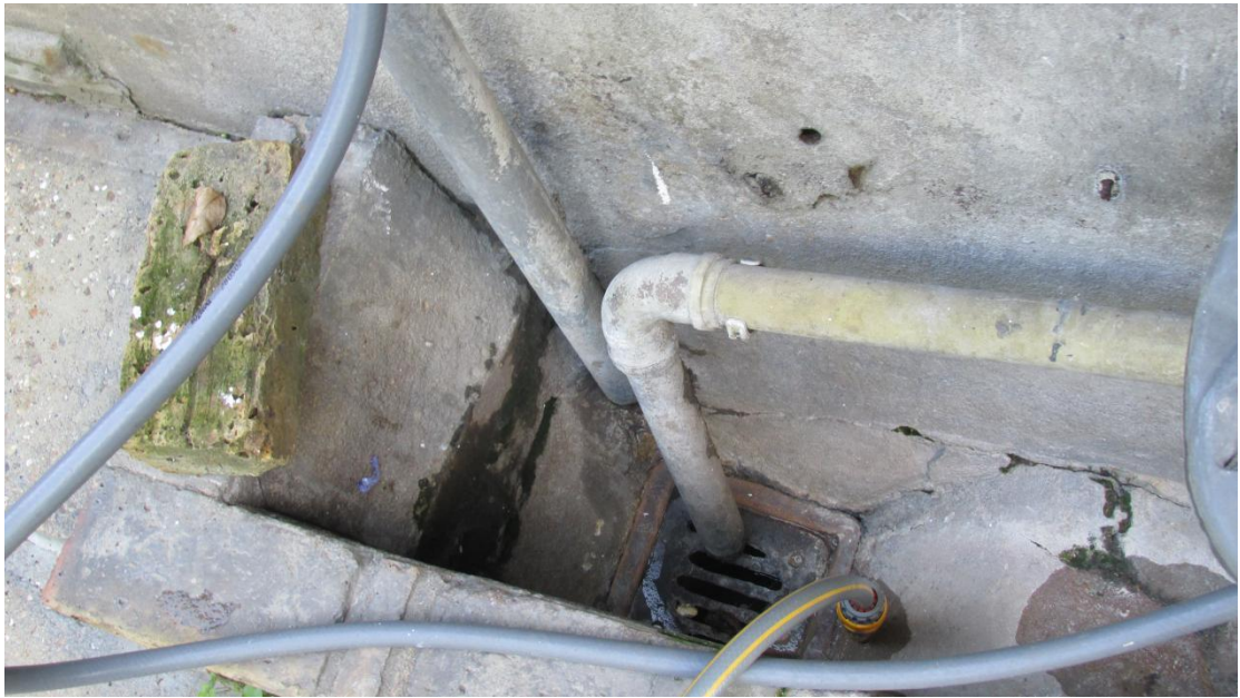
Rainwater gully at the rear
