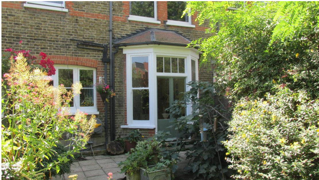
Rear bay timber windows
