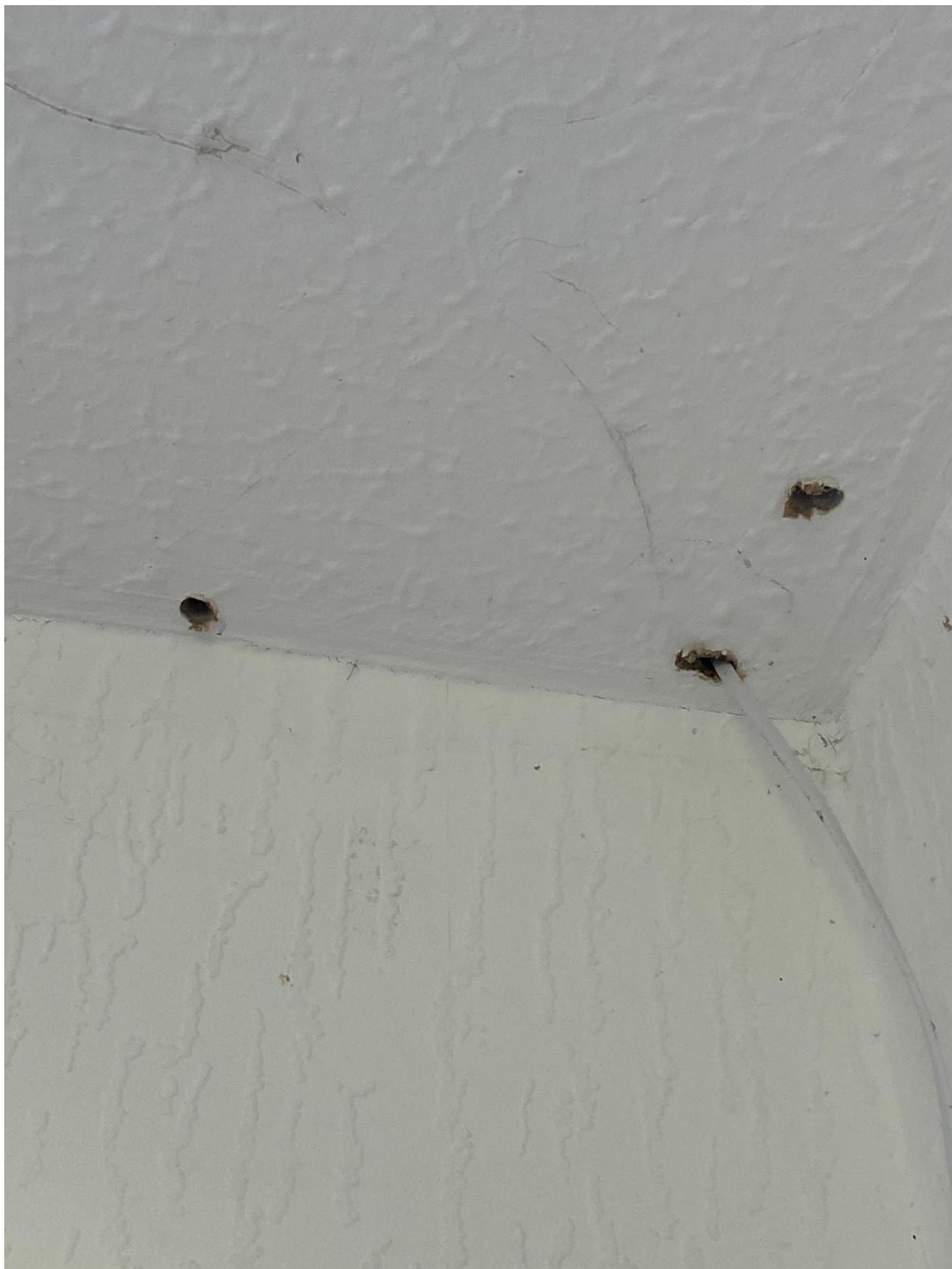
Ceiling in the rear utility room
