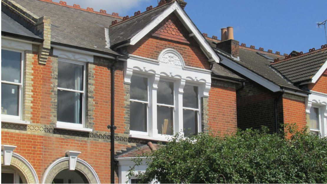
Front walls partially covered with clay tiles cladding
