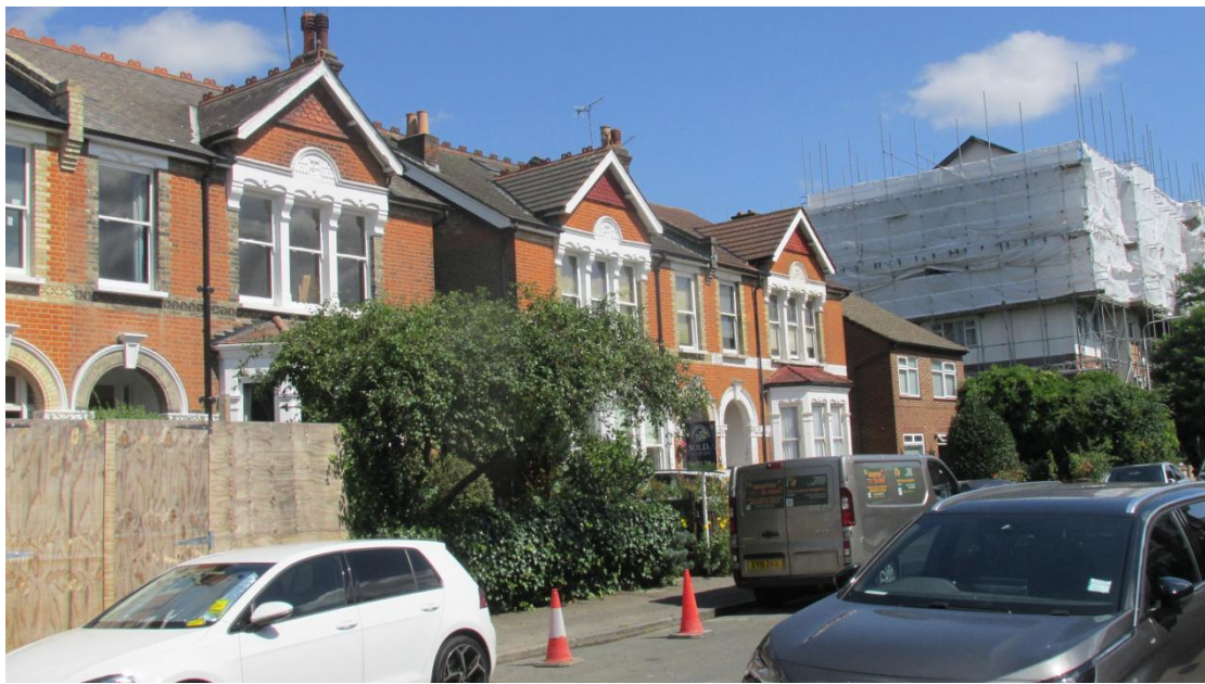
Front timber windows
