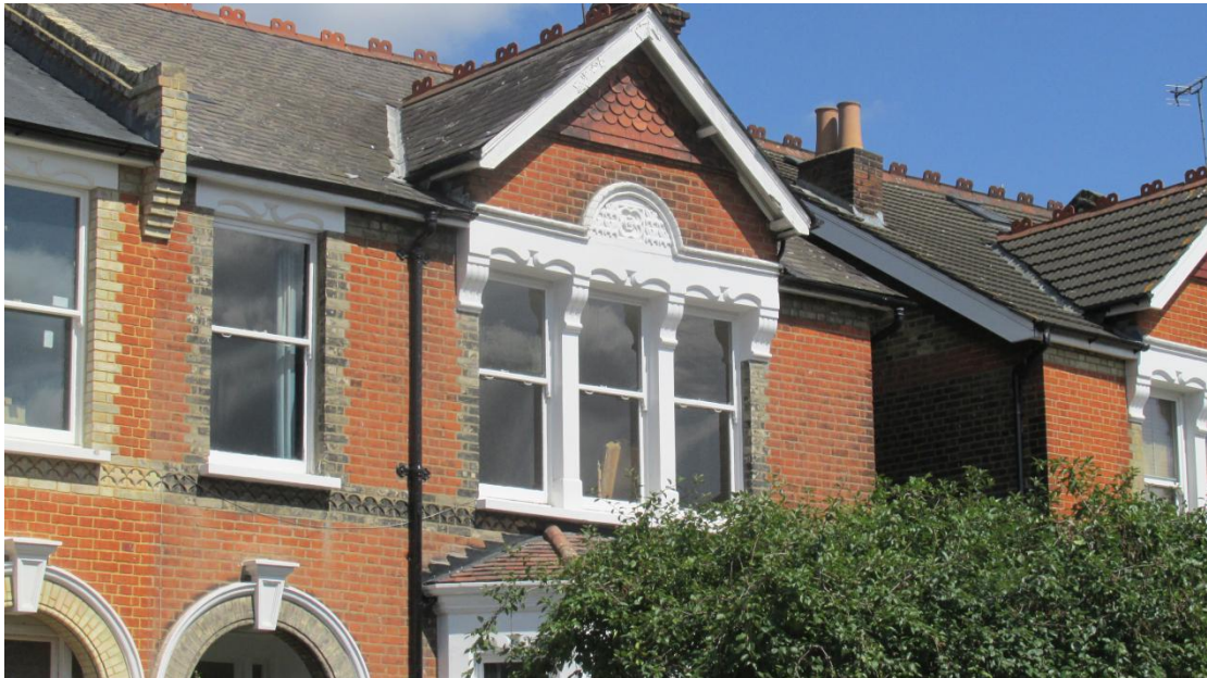
Gutters and downpipe at the front
