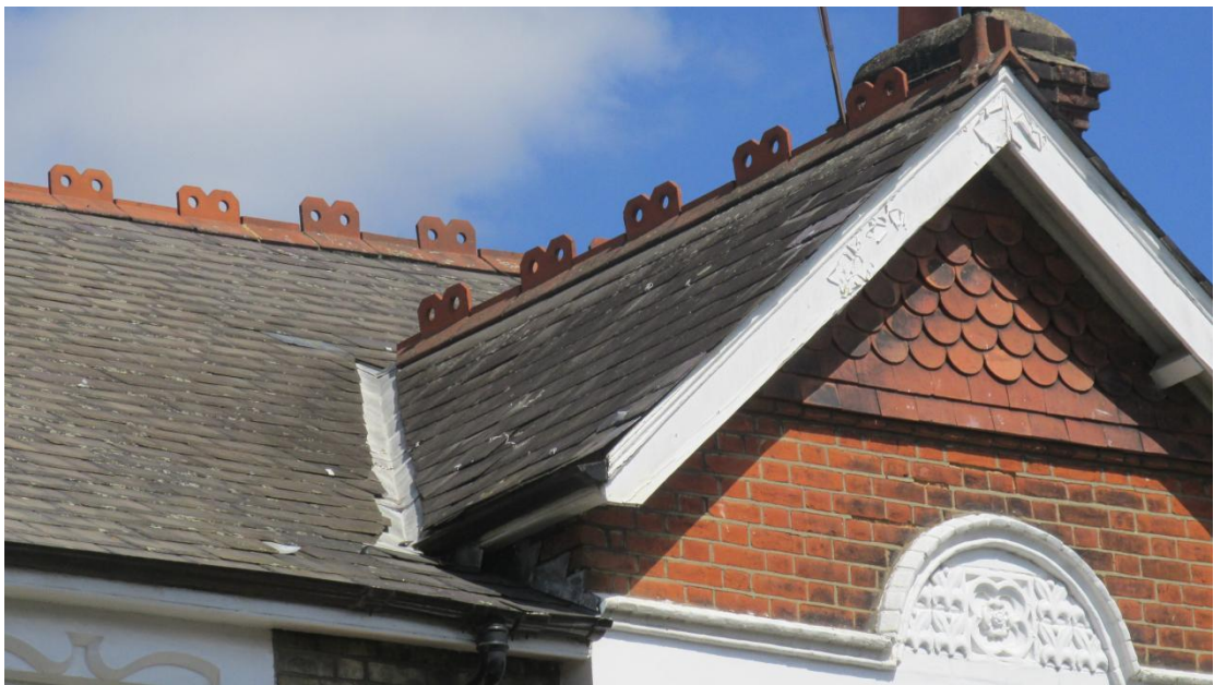
Roof on the front gable from left
