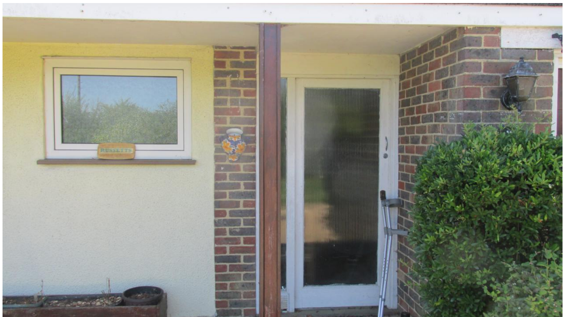
Front entrance door to the garages
