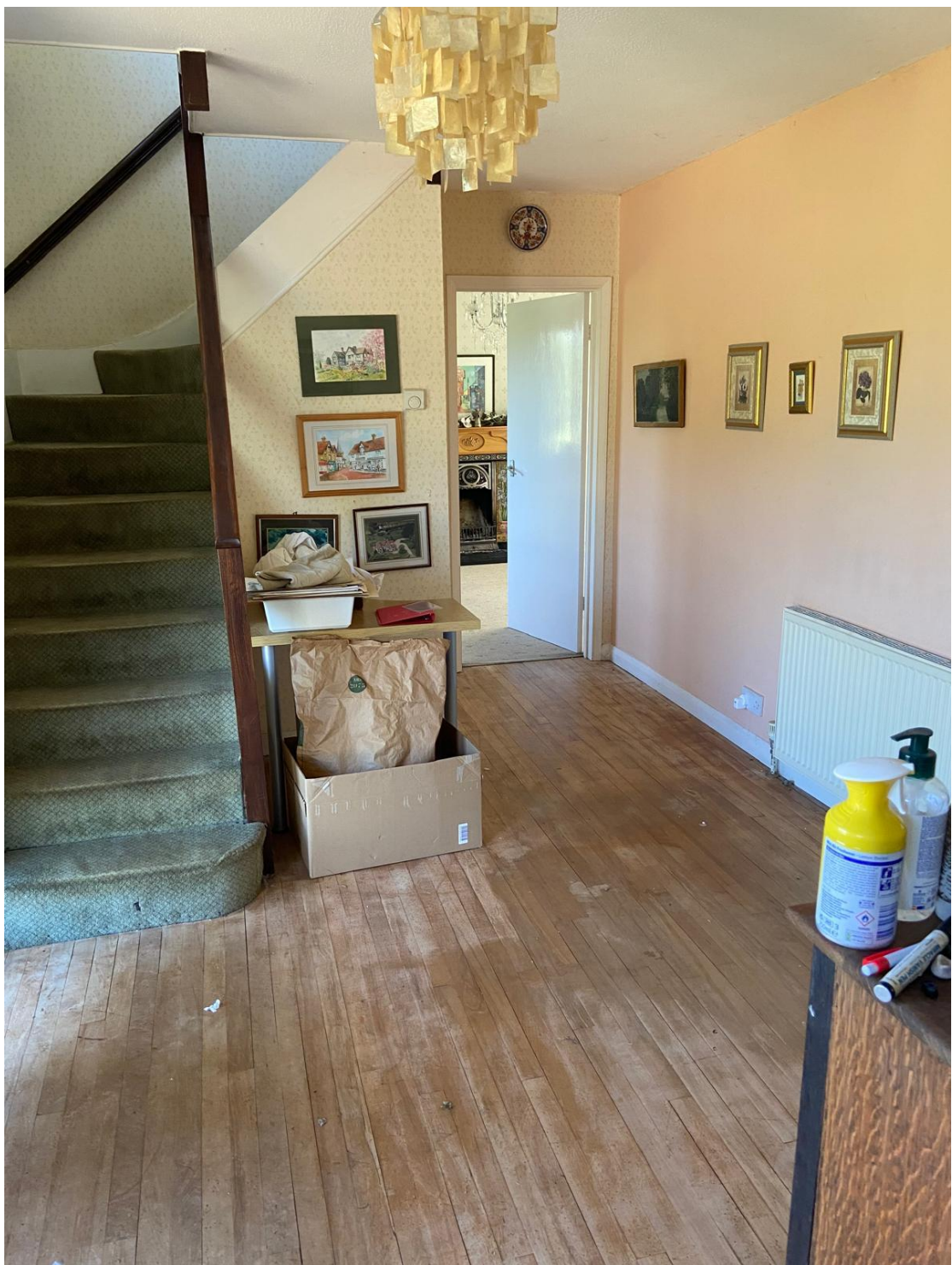
Floor in the corridor
