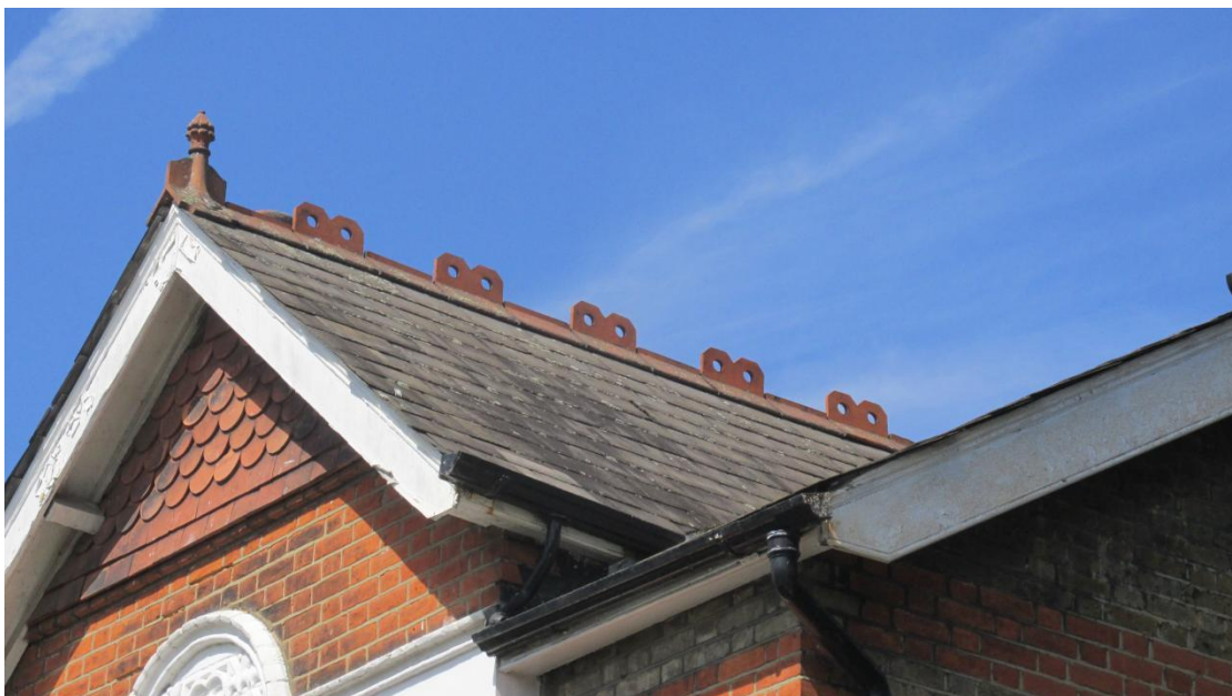
Gutters and down pipe at the right front
