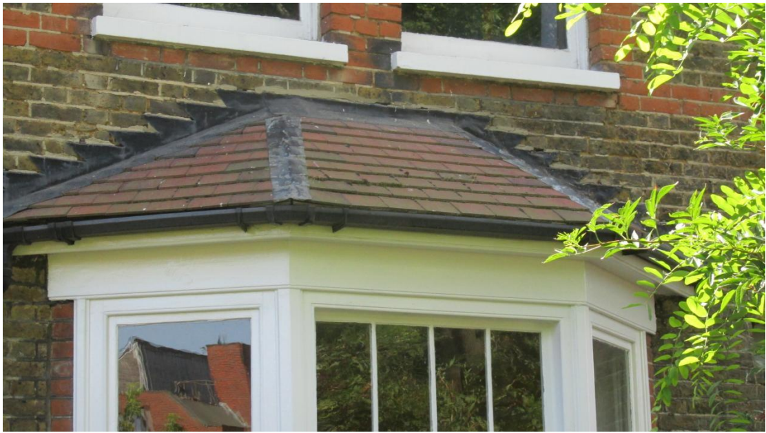
Roof on the rear bay window
