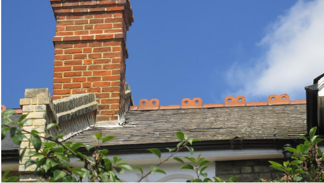
Roof covering from the front left
