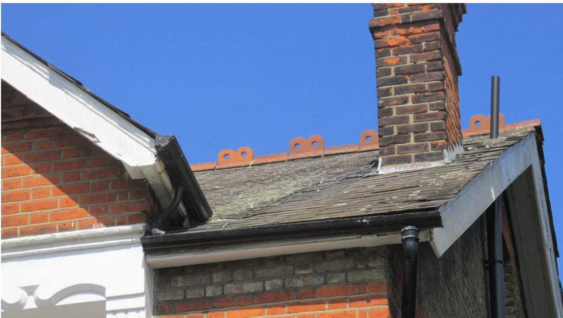
Right chimney stack flashing
