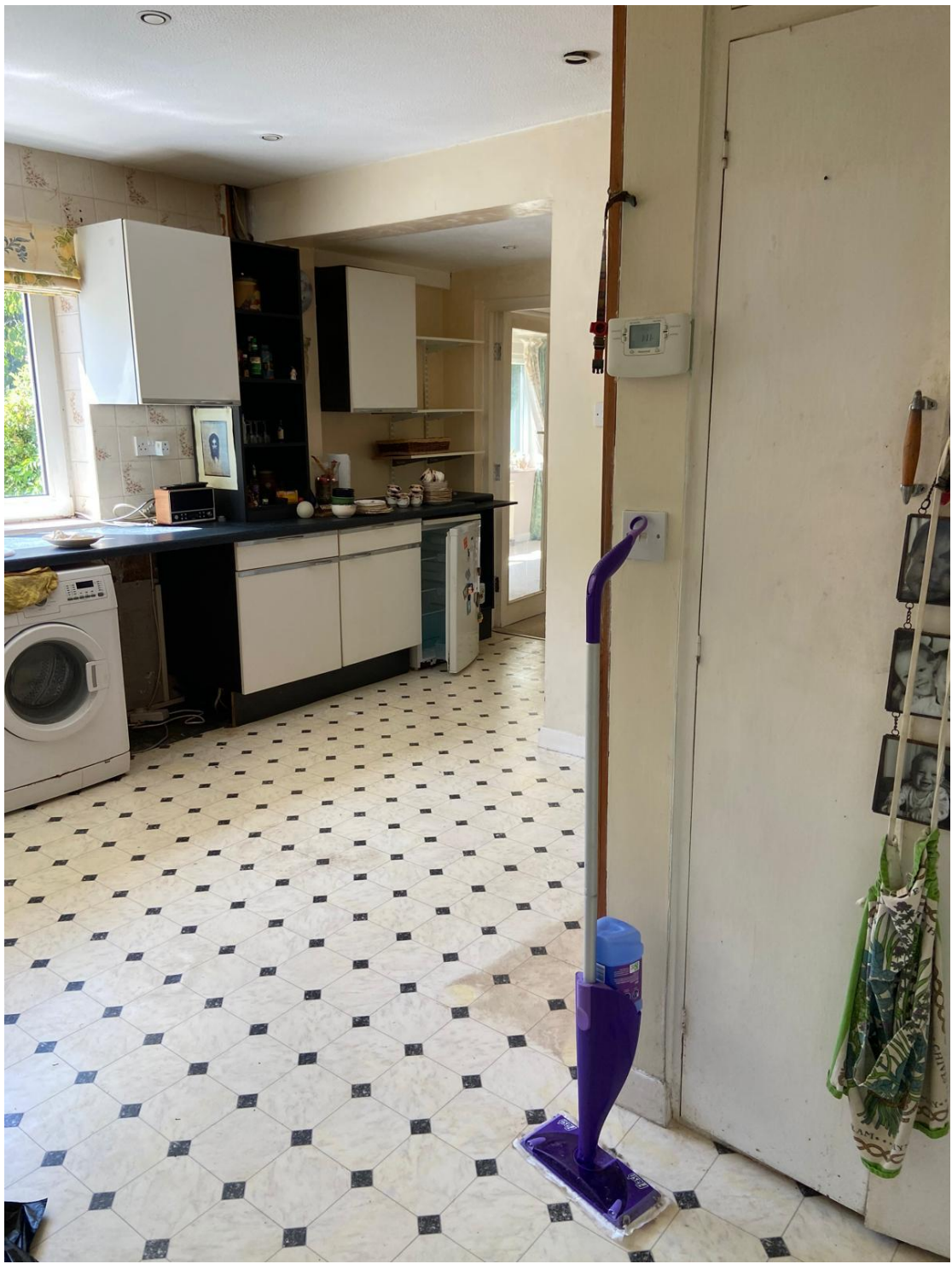
Kitchen floor covered with lino
