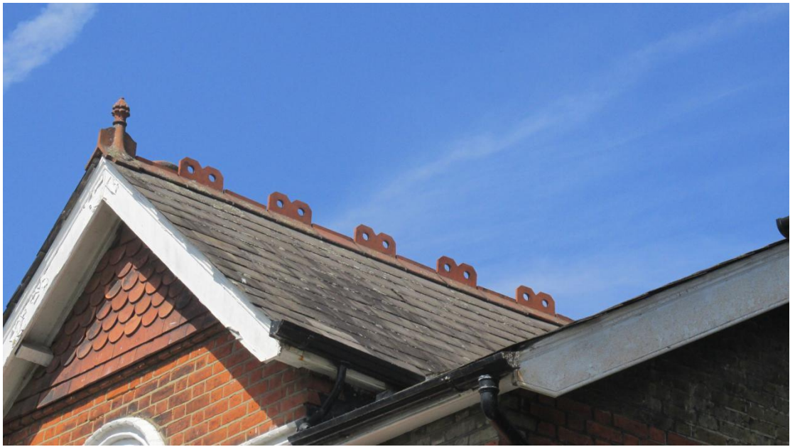
Front gable roof from the right
