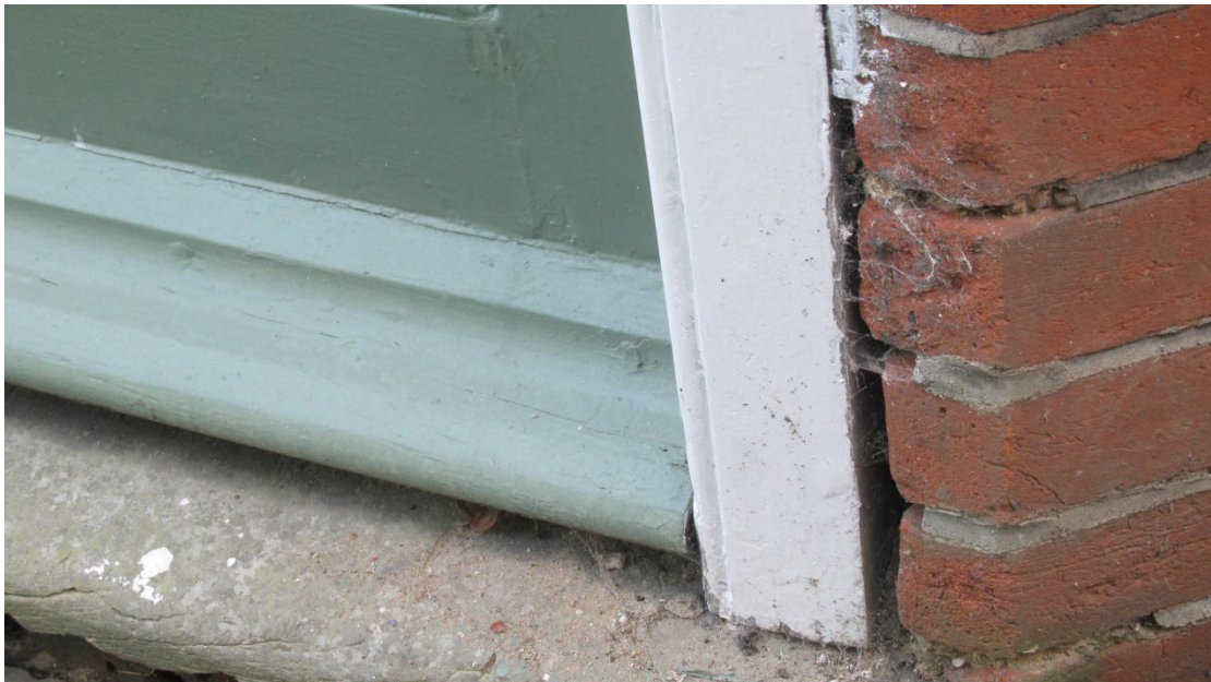
Rear wall near the door
