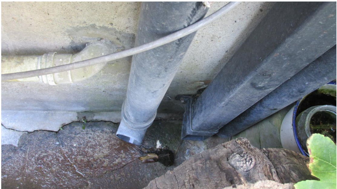
Rainwater pipe and gully at the rear
